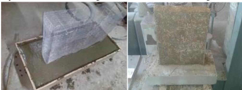
(a) Laying foundation and G.I. Wire mesh (b) Filling layers of earth and straw
