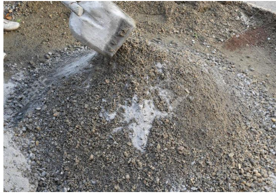
Figure 1 Mixing the Concrete Ingredients
