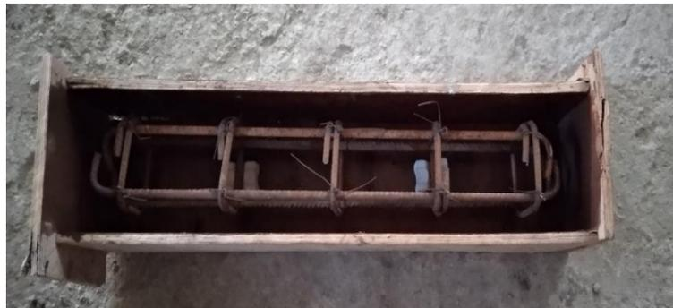
**Fig. 2.2 Steel Frame Used for Casting of Beam**
