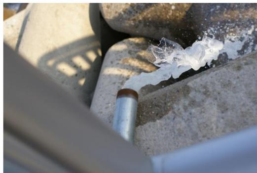
**Fig. 5; Outflow of Seawater through One of Multi-outlets**
